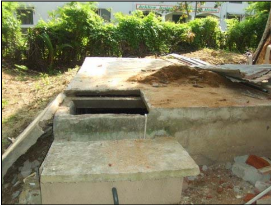
Underground water-storage for a school and orphanage in Weligama, Sri Lanka
